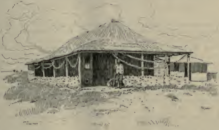
MR. WATERS' RESIDENCE IN TONGALAND—MADE OF WATTLE AND CLAY WITH THATCHED ROOF
